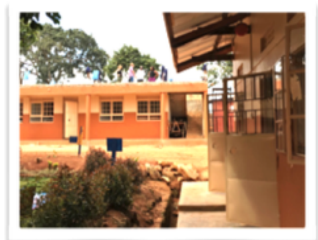
A partial view of the new classroom block: board members survey the campus from the second floor.
