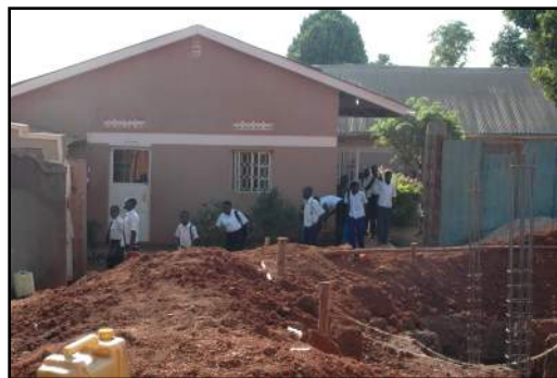
During construction, students still attend school in the other classroom blocks Alice and Mtaala constructed.
