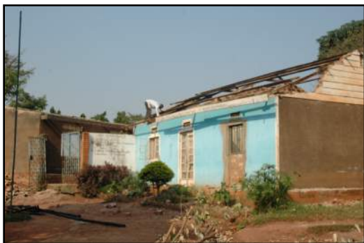
To make way for the new school building, demolition begins on Alice's former home, the house she had turned into a school for needy students.
